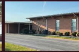
highland high school bonds were sold to fund the building of the first school in cherokee village. completed in 1964, highland high was built on land donated by john cooper, who also dedicated equipment and labor to its construction.
