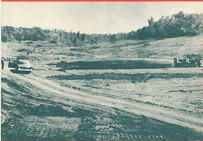
Earth-moving equipment shapes a lake.
